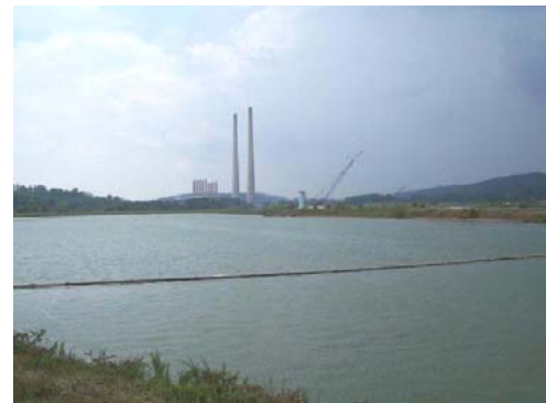
Figure 2: Typical Surface Impoundment (Ash Pond)
