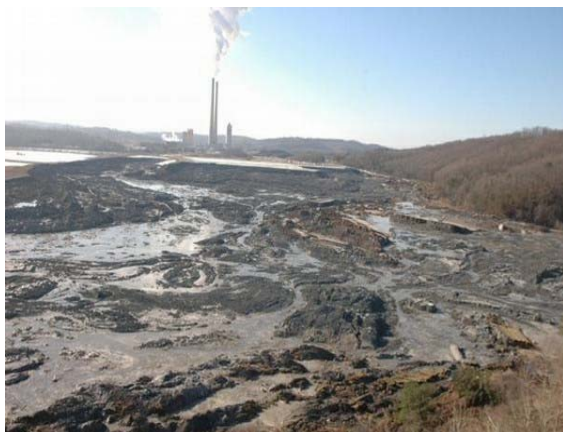
Figure 3: Typical Surface Impoundment after berm failure
