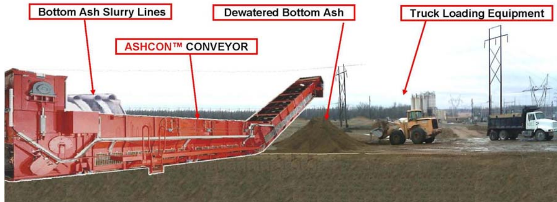
Figure 12: ASHCON™ Remote Submerged Scraper Conveyor Retrofit
