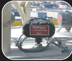
Measuring dry feed supplements in bulk storage silos.
